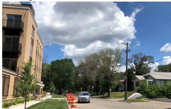
Figure 2: Liffey Apartment Building at Snelling & Carroll Avenue
